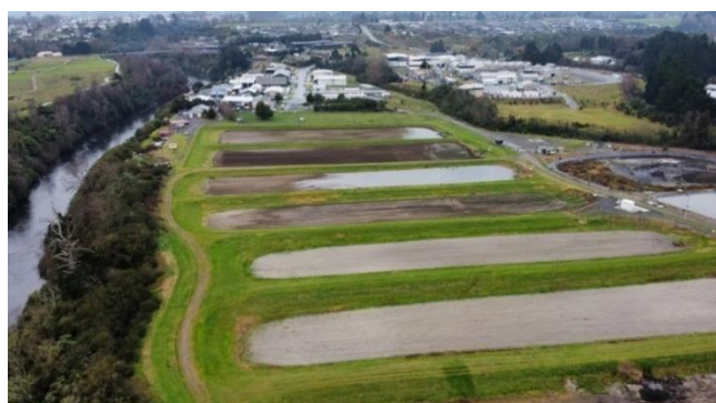
Figure 2 - Rapid Infiltration Beds in the forefront.
