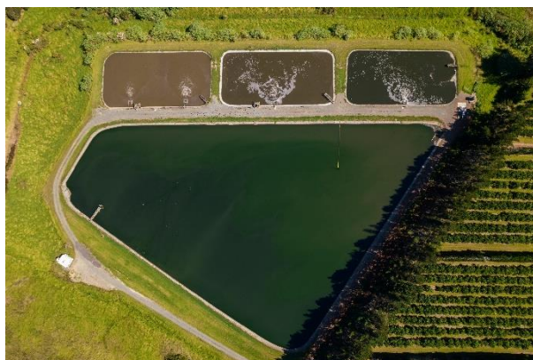
Figure 1. Taipā WWTP (image owned by Far North District Council)
